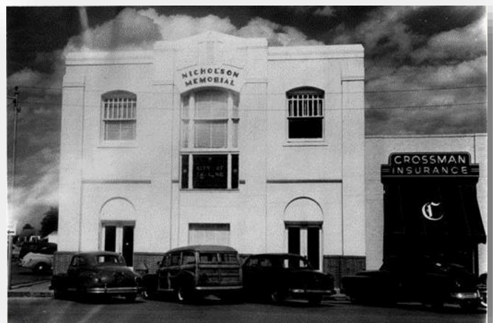
This image, ca. ***, shows the now demolished east side of the square with Nicholson Memorial Hall (formerly Citizens National Bank) and Crossman Insurance.
